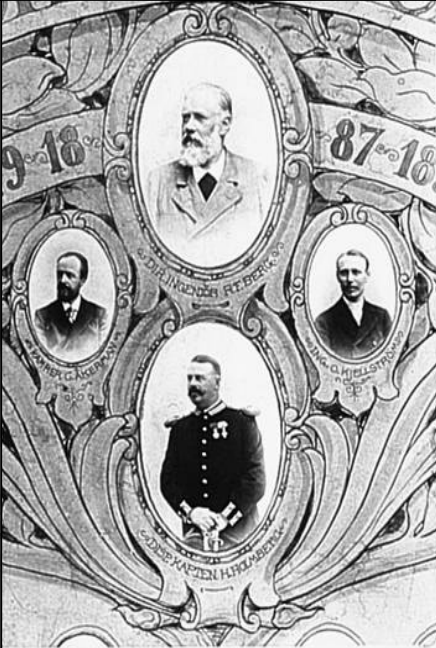
1887 AB Skånska Cementgjuteriet founded by R.F.Berg
